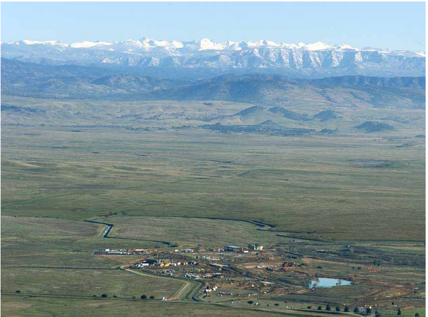
The Sierra Nevada northeast of the campus site during construction, 2004.
