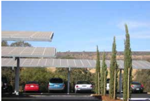
Solar Parking Shades
