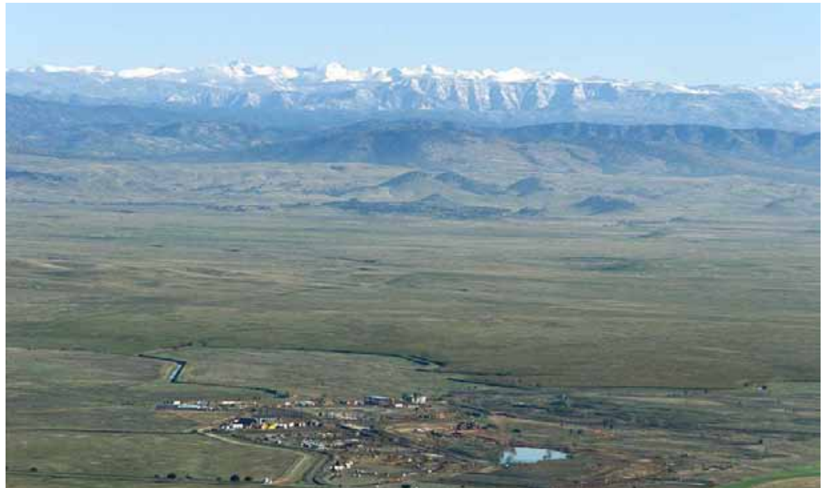
Northeast view of campus construction, 2004. The Sierra Nevada and permanently protected wetlands edge the northern and eastern campus boundaries.
