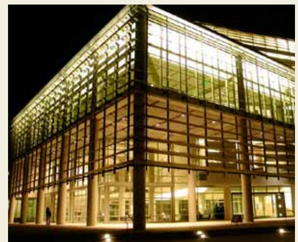
Internal light creates a lantern effect at night.
