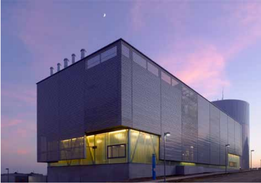
Central Plant, LEED Gold
