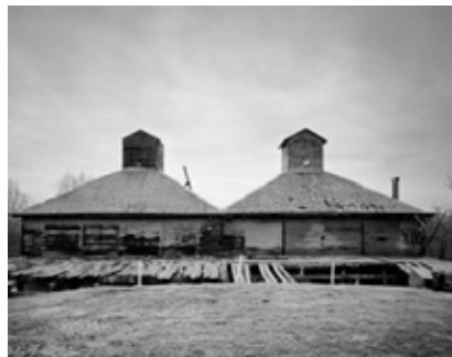
Abandoned Hop Kilns.
