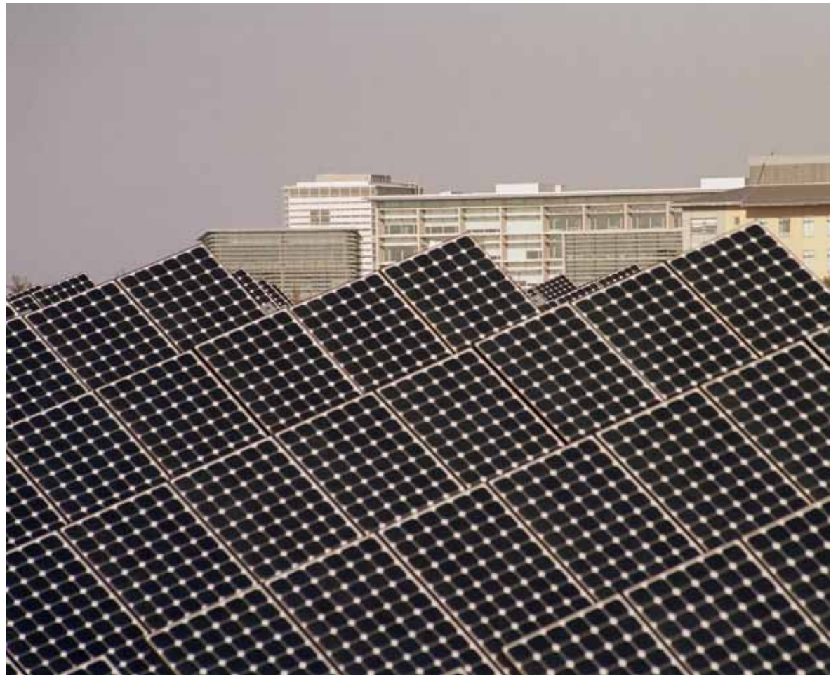
UC Merced's 1 megawatt solar array provides 20% of the campus energy needs, exemplifying the campus' ability to maximize the potential of its setting.
