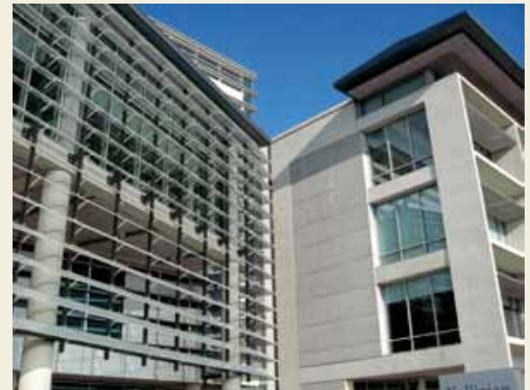
Glass, steel and concrete composed in utilitarian forms evokes Central Valley agricultural industrial structures.
