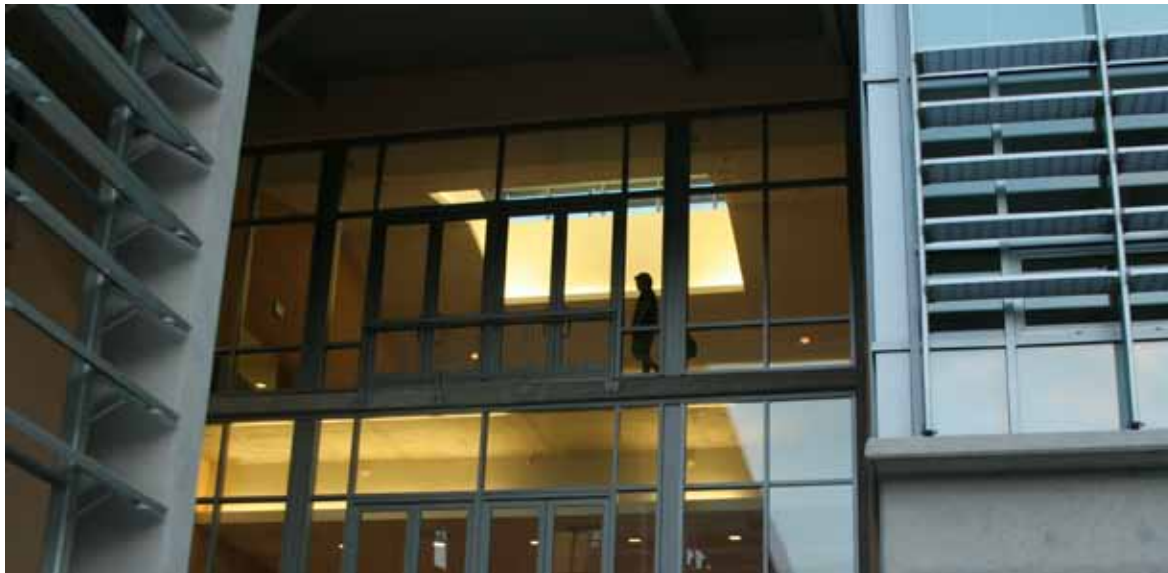
The Academic Core exemplifies the use of concrete, glass and steel.
