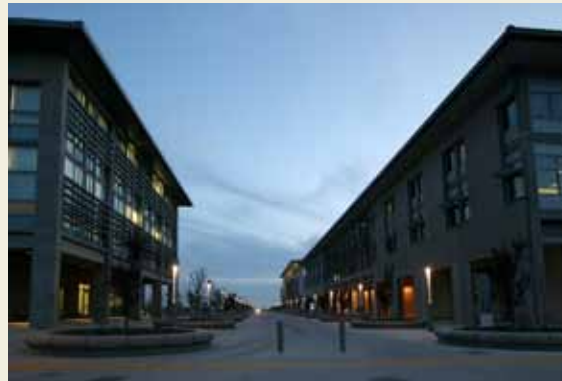
Science and Engineering 1 and Classroom Office Building
