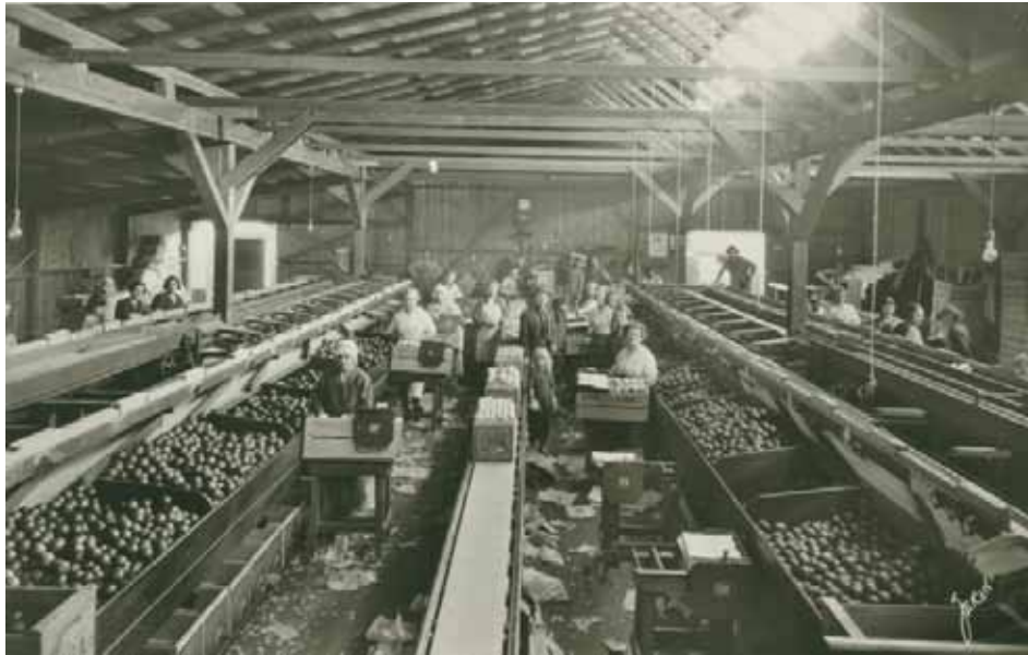
Orange Packing Shed, Kern County, 1922.
