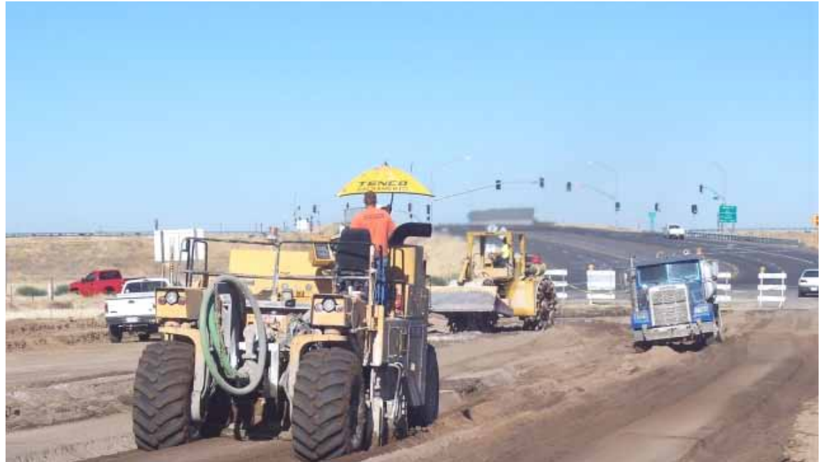
Campus Parkway, Phase 1 construction at Highway 99. The first segment of the Campus Parkway that will connect the campus to Highway 99 is in progress. Construction of Phases 2 and 3 are dependent on state, local and federal funding.
